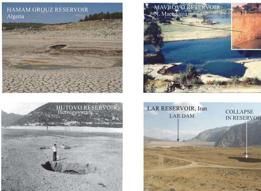
Fig 5. Collapses occurred during first filling or as consequence of reservoir operation.
